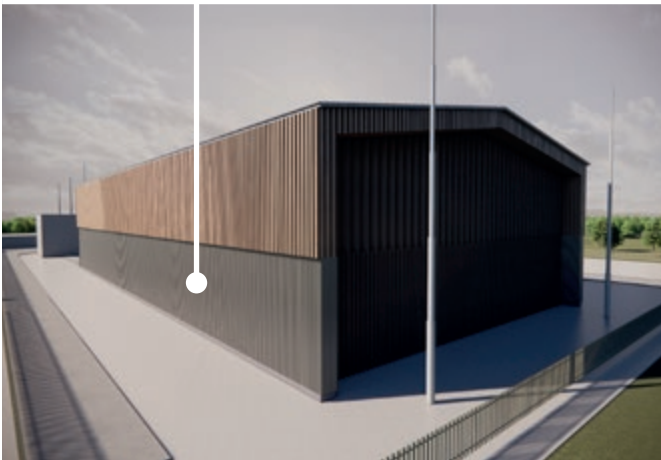
Lower level metal cladding found in OCS infrastructure (e.g. greys)
